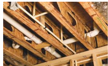
Wooden I-Joists with cutouts for piping and other system components.
